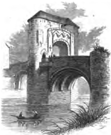
RAGLAN CASTLE BRIDGE.
